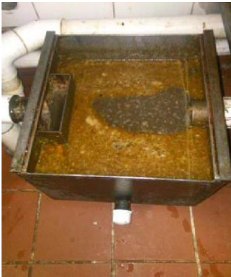
Trap FOG Accumulation
