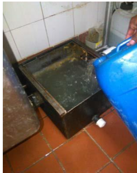
Cleaning/Disinfection of Trap
